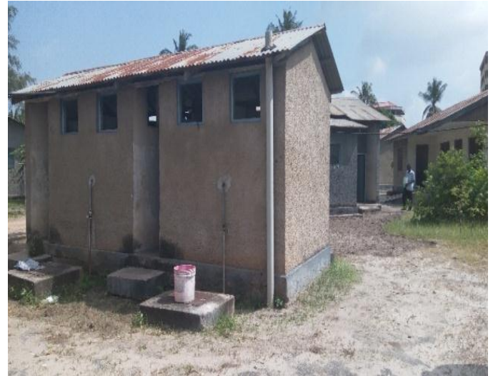
Figure 16: Outdoor toilets Source: fieldwork , 2017
